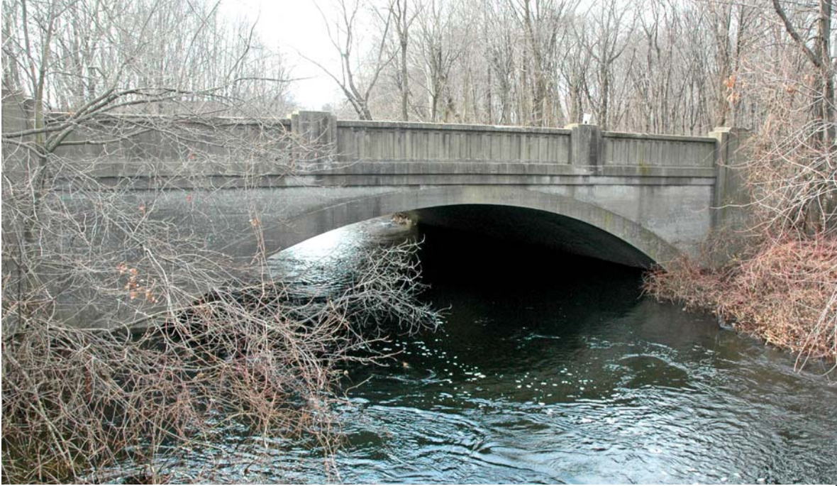
Franklin Street Bridge. 2008 photo.
