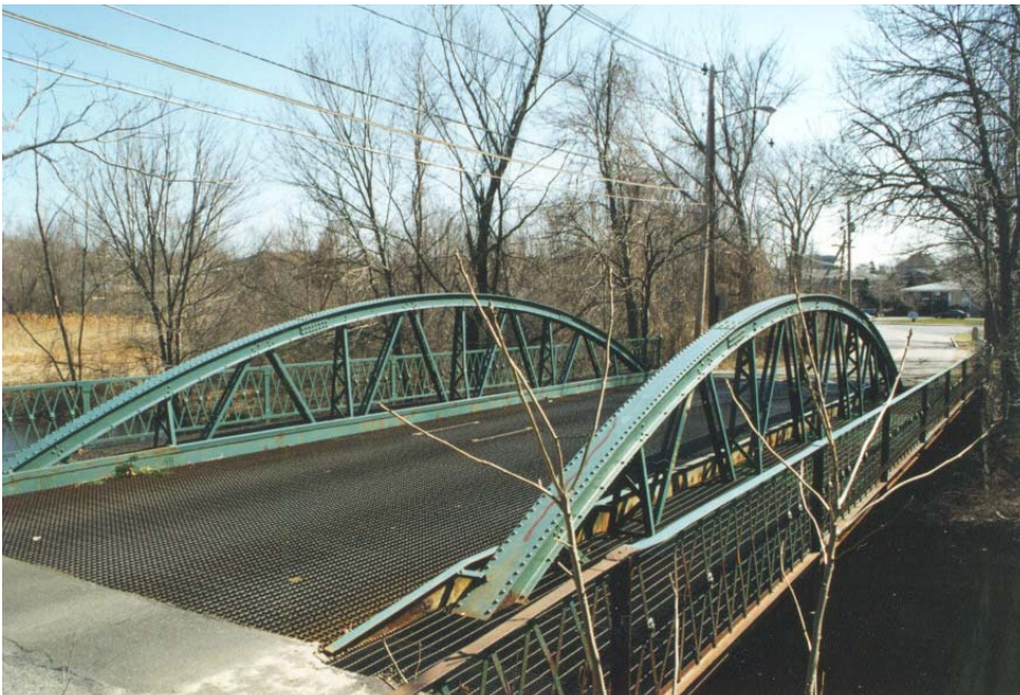
Figure 1. The Main Street Bridge, circa 1995.
