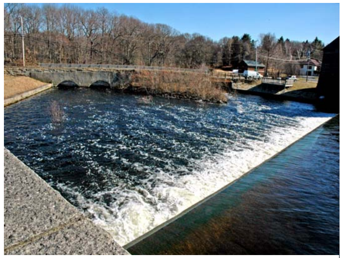
Photo 8. View of causeway looking east from top of spillway of dam. The bridge at the south end of the causeway can be seen in the right background.
