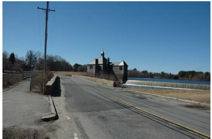
Photo 7. Causeway looking south. Stone arch bridge is on the near end of the causeway. The dam is to the right and the footbridge is to the left.
