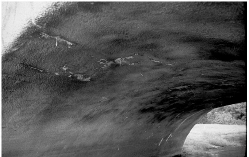
Figure 3. View of bottom of one of the arch barrels. 1977 photo.
