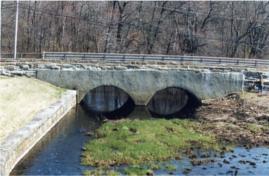
Figure 1. Upstream view of the Winter Street Bridge over the Sudbury River. Bridge built in 1700s. 1995 photo. Causeway extends from both ends of the bridge. Stone wall and banking in left foreground added in the 1870s.
