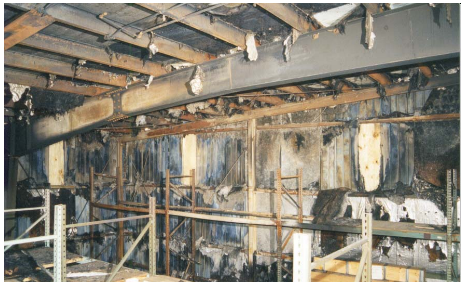
Figure 4. View of rigid frame on Line 8, west of the ridge. In the background is the framing at the end wall on Line 9.
