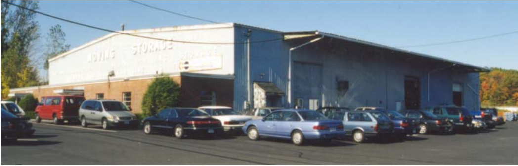
Figure 1. View of south and east sides of moving company warehouse.
