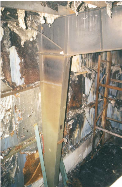
Figure 3. View of rigid frame at grid location A-8.
